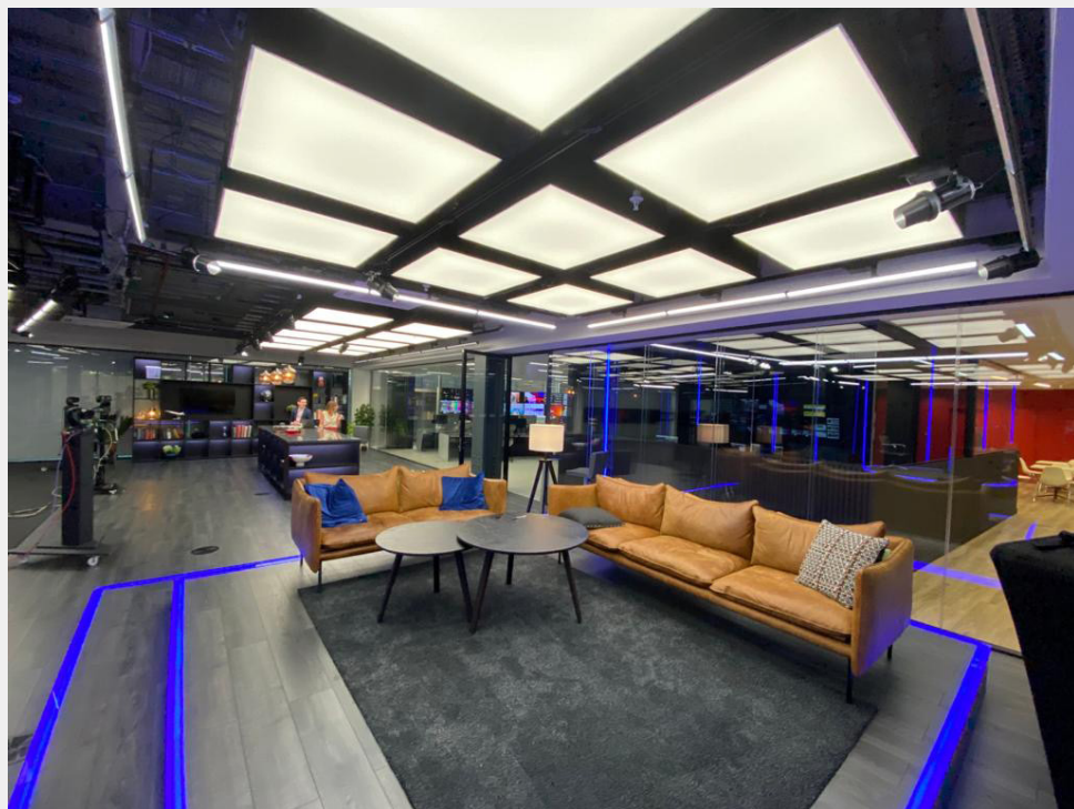
B&S Track Lights installed at GB NEWS
